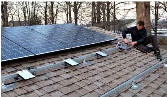
A microinverter system being installed
